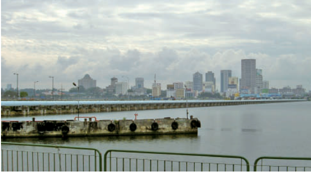
Pipelines conveying water from Malaysia to Singapore.
