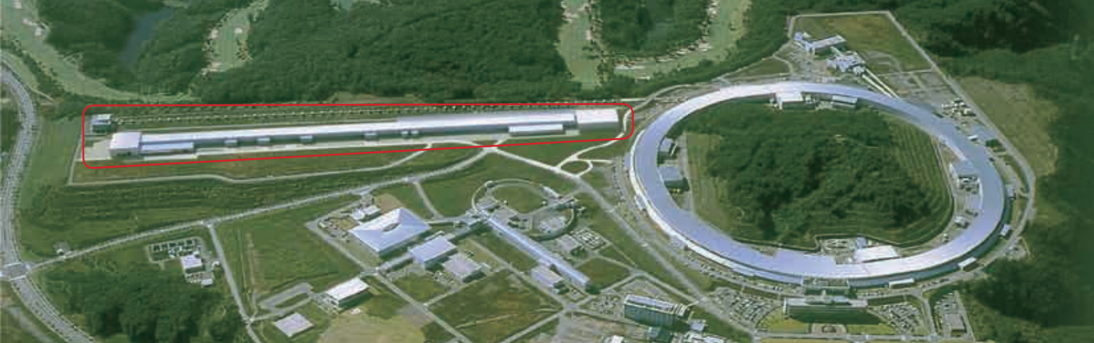
Aerial photo of the construction site
